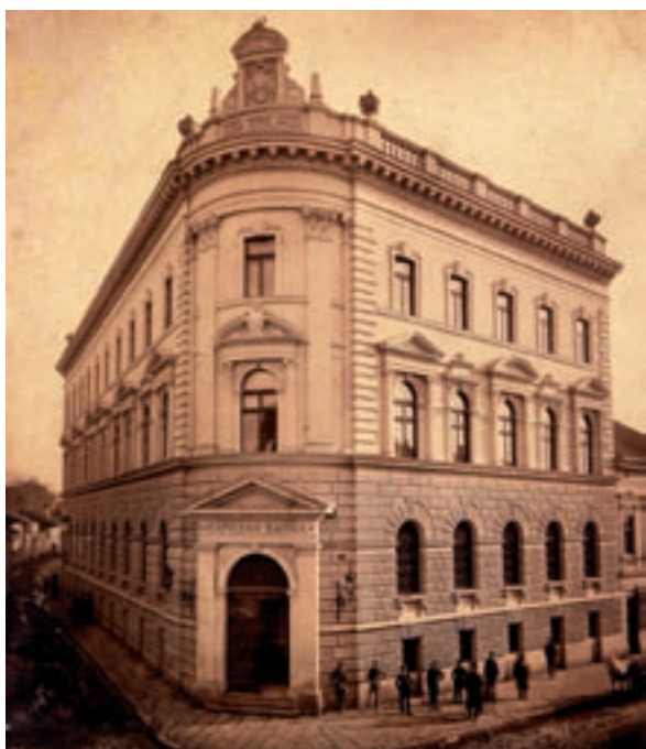
The Old National Bank of Serbia Building” dating back to the end of XIX century
