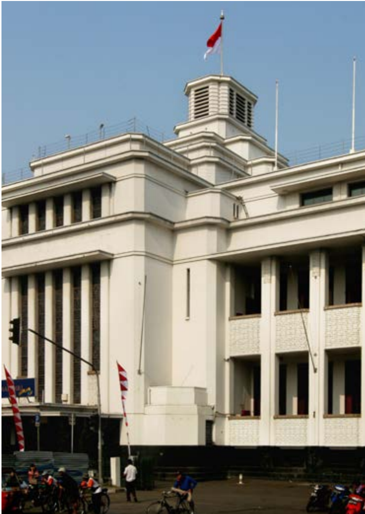
One of the three ventilation towers giving the building a distinguishing silhouette (copyright: ABN AMRO Art & Heritage)
