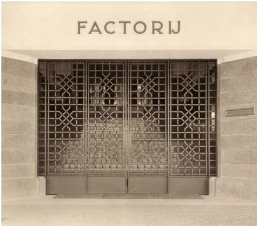
The gate in the main entrance allowed for extra ventilation throughout the banking hall. (copyright: ABN AMRO Art & History)
