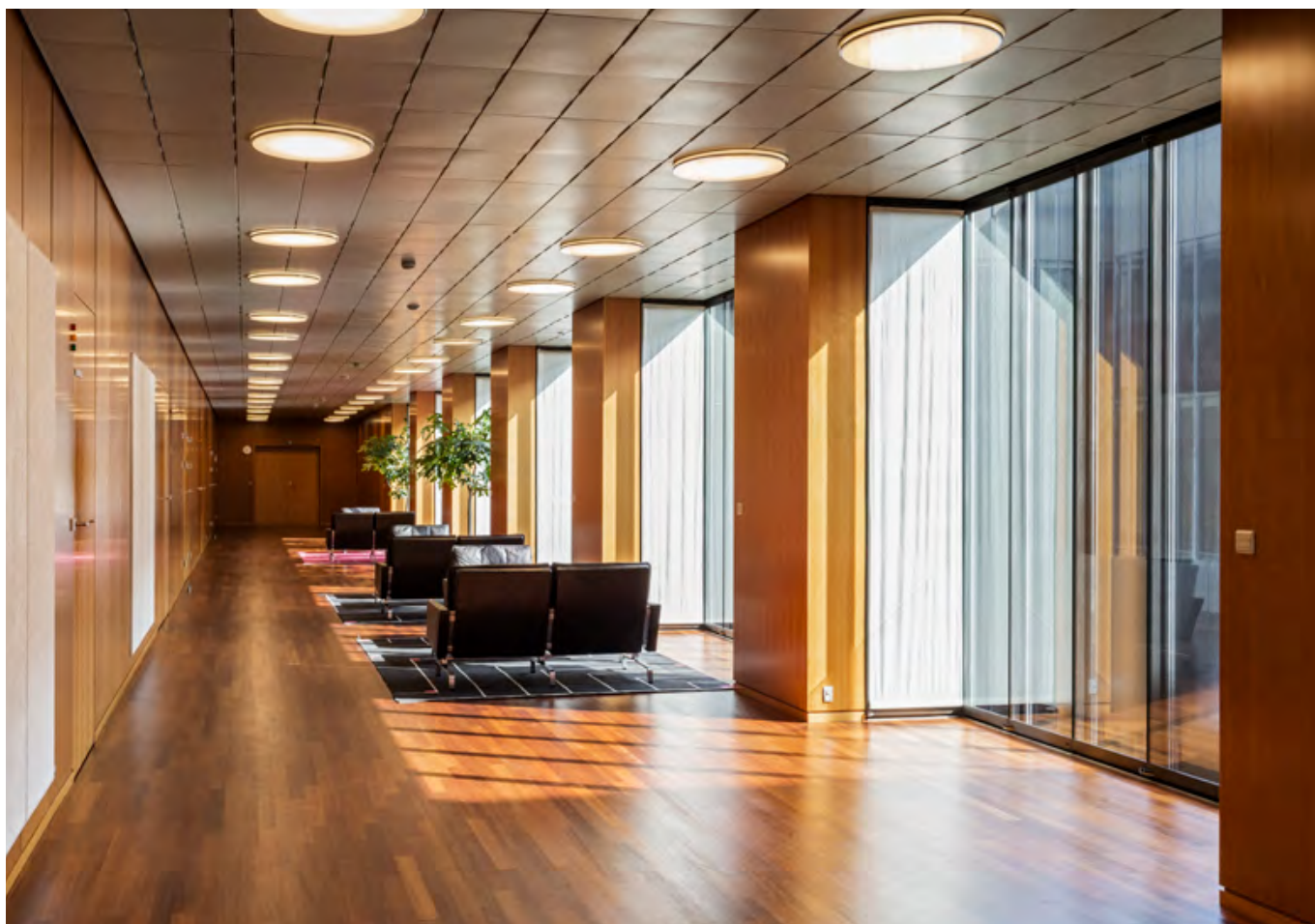
Corridor outside the governor's office. Walls clad in knotless Central European pearwood and floors in West African Doussie-wood – both of which materials are used consistently throughout much of the bank's interior
