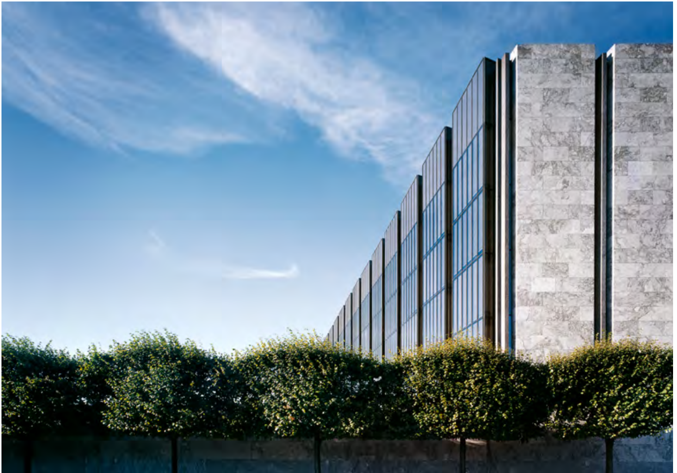
Two types of façades: The open glass-faced bays and the closed marble fronts, divided up into rectangular forms
