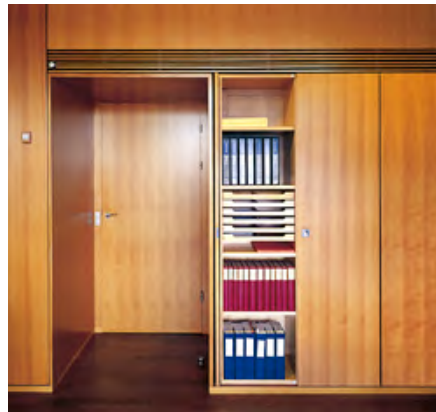
A versatile, pearwood-veneered storage and partitioning unit serving both the corridor side and office side with combinations of coat-rack, cabinet, drawer and shelving modules
