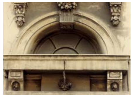
Details of neoclassical buildings in Athens
