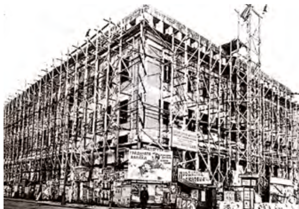
The building under construction - BNB Archives
