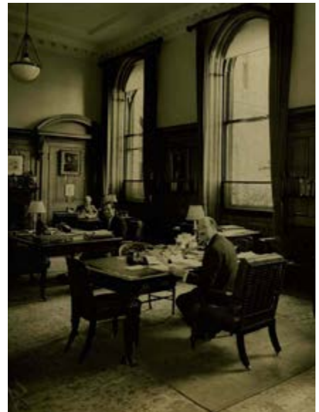
The Partners' Room in the second New Court (c.1960)
